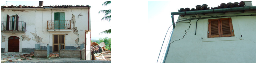
Fig. 1. Castelnuovo di San Pio delle Camere, L'Aquila, Italy (image by author). (a) Effects of the earthquake on the façade of a residential building in stone and masonry; (b) Effects of the earthquake on the façade of a residential building in stone and masonry.
