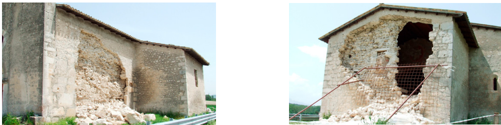
Fig. 2. San Pio delle Camere, L'Aquila, Italy (image by author). (a) Effects of the earthquake on the side wall of a stone church; (b) Effects of the earthquake on the end wall of a stone church.
